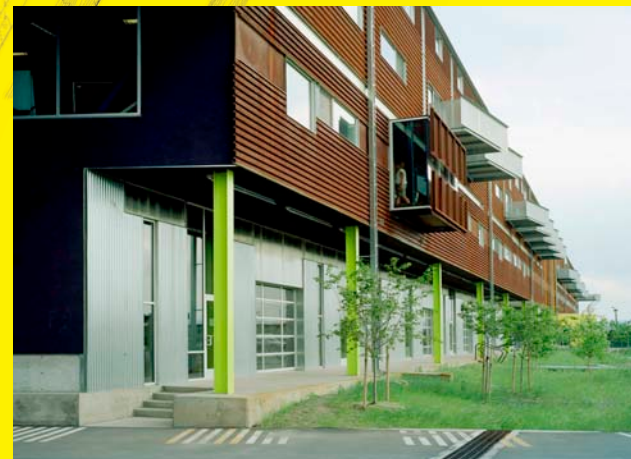
A shaded Walkway past business entries tucks under the West facade. Galvanized plank "bridges" cross over the landscaped PLD (porous landscape detention) drainage swale.
